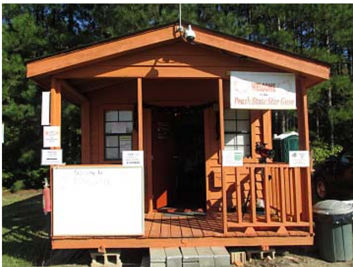
The Check-in Building at the PSSG
